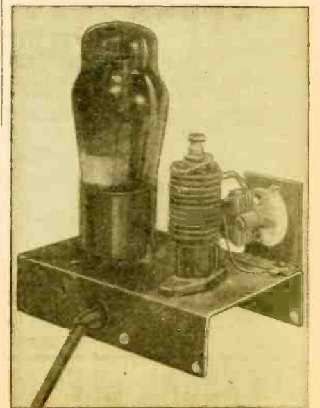
Subchassis holds the transmitting oscillator.
